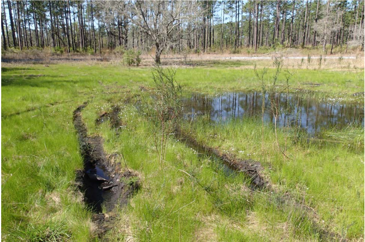
Figure 19. Vandalism at Pond 18, with 4x4 truck ruts throughout the wetland basin. Spinning tires created deep ruts and penetrated to the rubber liner, and punctured the liner in two places.
